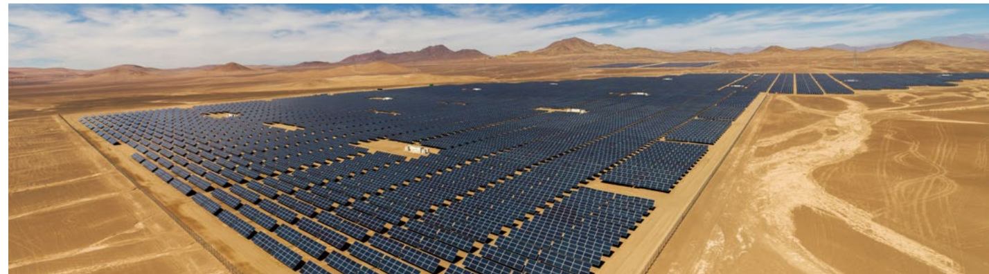
📍 The Chañares plant in Chile has an installed capacity of 40 MW and can generate up to 94 GWh per year. © Enel Group
